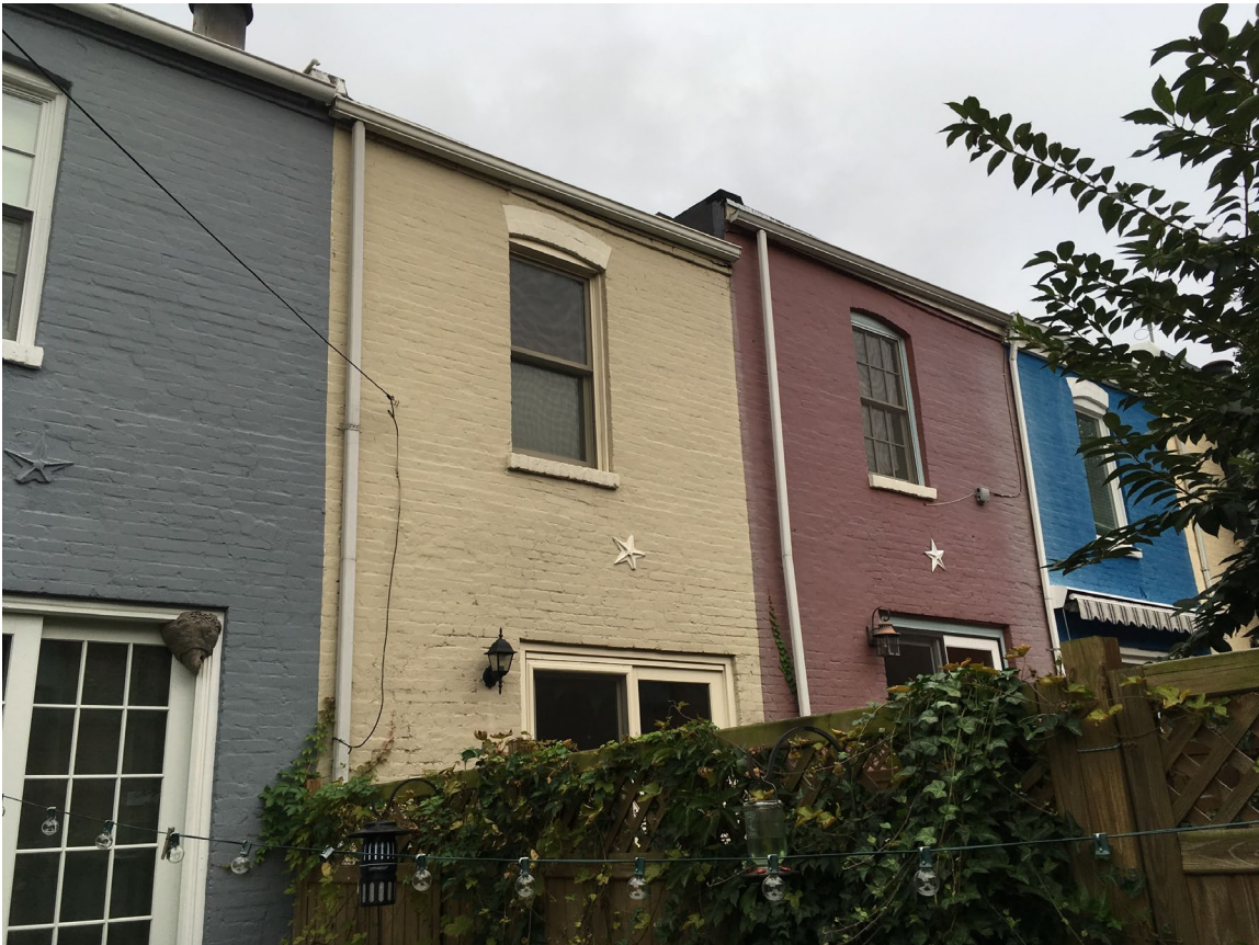
REAR VIEW LOOKING SOUTH
